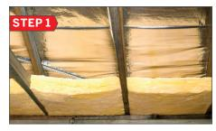
Push insulation out towards the eaves so the end of the first segment is 50mm into the top plate. Leave a minimum 20mm air gap between insulation and sarking membrane or roof material.
