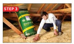
Ensure insulation ends are butted firmly together so there are no air gaps. To fill in any gaps trim insulation and use offcuts.
