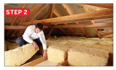
Lay insulation between ceiling joists using the poker to push them into limited access areas. Do not leave any gaps between the insulation and ceiling joists.
