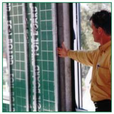
MOTOROLA OFFICE BUILDING - Here we demonstrate how FOILBOARD® INSULATION PANEL is applied to concrete structures using Beta-Fix adjustable clips and standard Rondo firring channel.
