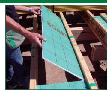
FOILBOARD® INSULATION PANEL is being used in conjunction with the FOILBOARD® FLOOR SADDLE during the construction process. Note the ease of application.
