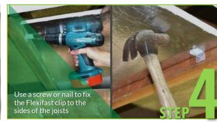
Embedding the spikes of the Flexifast clip into the FR-EPS core secures the Foilboard® GREEN panel in position ensuring quick and easy installation
