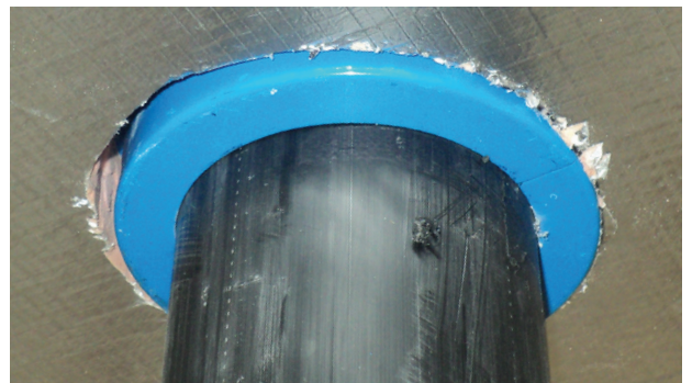
Figure 7 Penetration example - Kingspan Kooltherm ® K10 G2 Soffit Board installed tight around the fire collar and HDPE service pipe.
